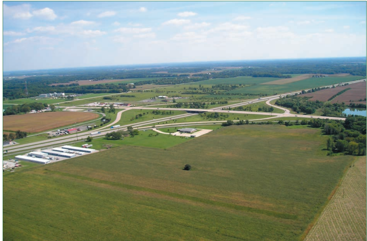
I-55/IL Route 143 Intersection
